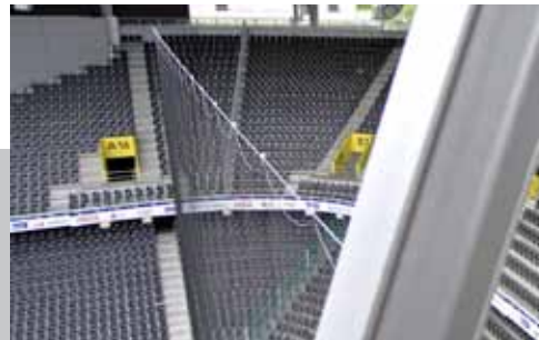
Elaborated: minimal-invasive installation with multi-safety device
