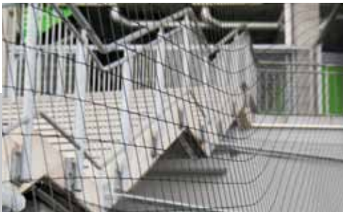
Prevents pyro-smuggling: customised netting at stairways
